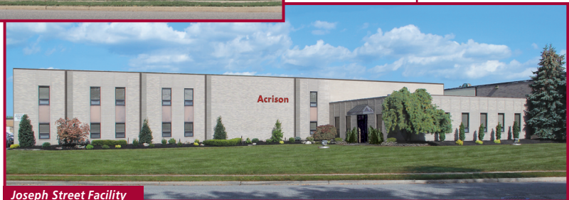
Joseph Street Facility Moonachie, NJ USA
