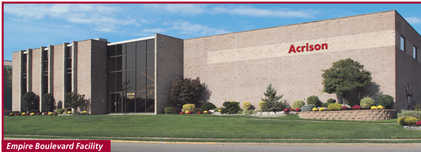
Empire Boulevard Facility Moonachie, NJ USA
