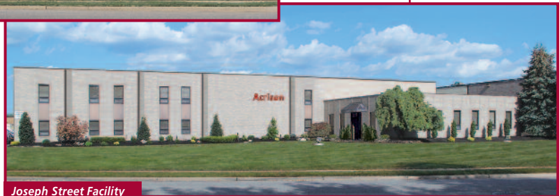
Joseph Street Facility Moonachie, NJ USA
