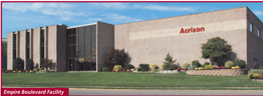
Empire Boulevard Facility Moonachie, NJ USA
