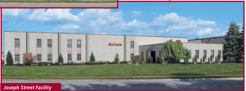
Joseph Street Facility Moonachie, NJ USA
