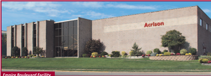
Empire Boulevard Facility Moonachie, NJ USA
