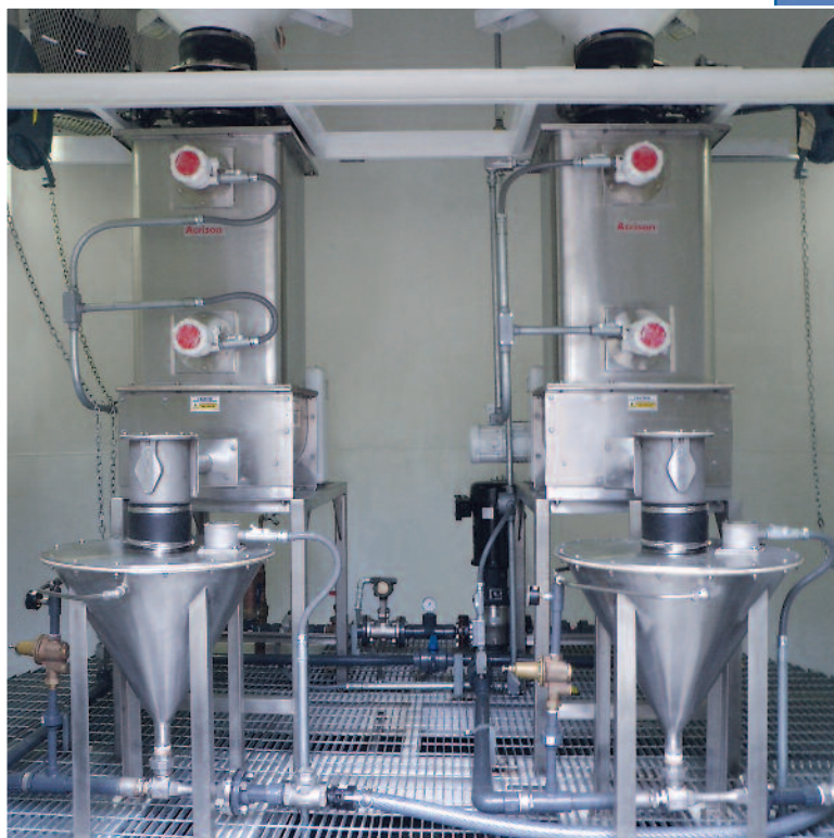
The exterior and interior of a typical skirted Silo. A portion of the applicable Acrison Equipment can be seen installed inside the skirted bottom.
