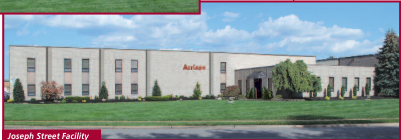
Joseph Street Facility Moonachie, NJ USA
