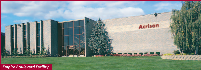
Empire Boulevard Facility Moonachie, NJ USA
