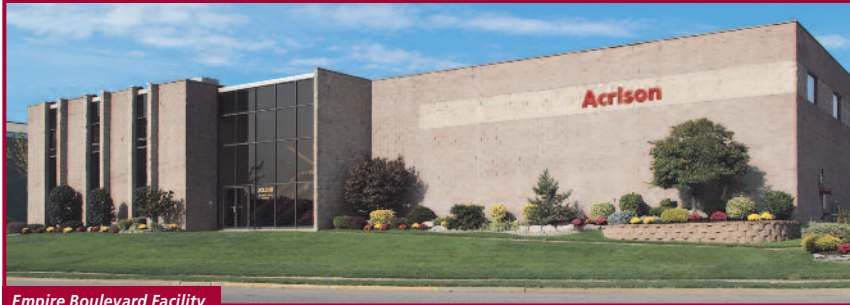
Empire Boulevard Facility Moonachie, NJ USA
