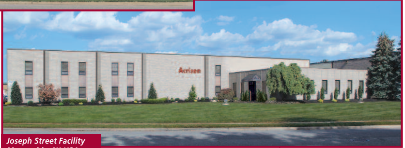
Joseph Street Facility Moonachie, NJ USA
