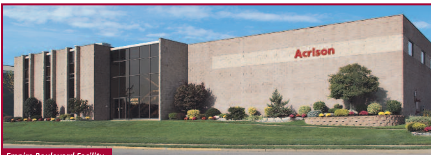
Empire Boulevard Facility Moonachie, NJ USA
