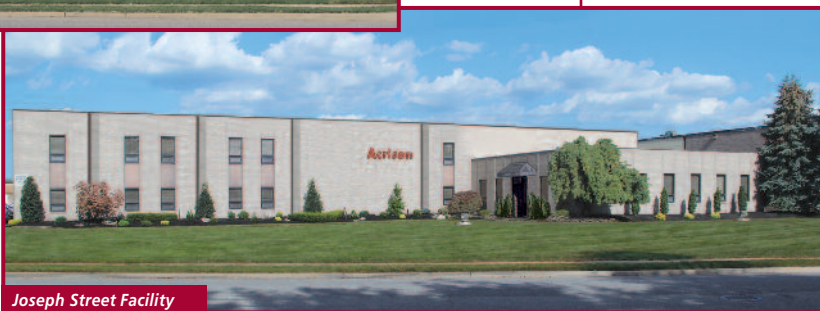
Joseph Street Facility Moonachie, NJ USA
