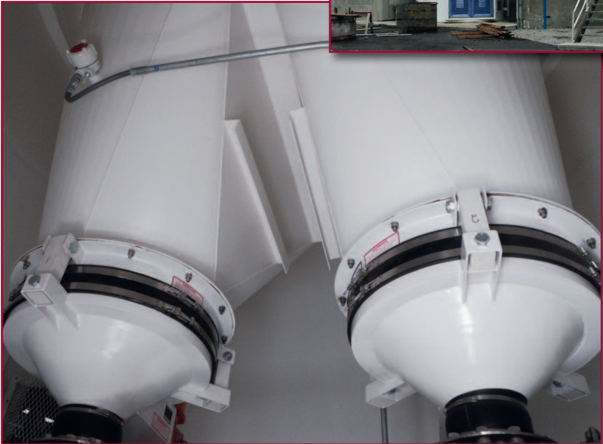
Top: A skirted silo with a reverse air-clean dust collector used for a municipal lime storage and feeding application.
