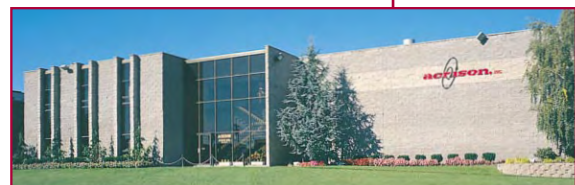
Empire Boulevard Facility Moonachie, NJ USA
