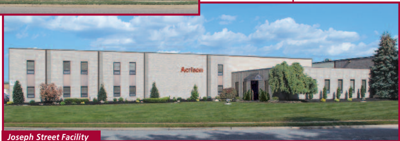
Joseph Street Facility Moonachie, NJ USA
