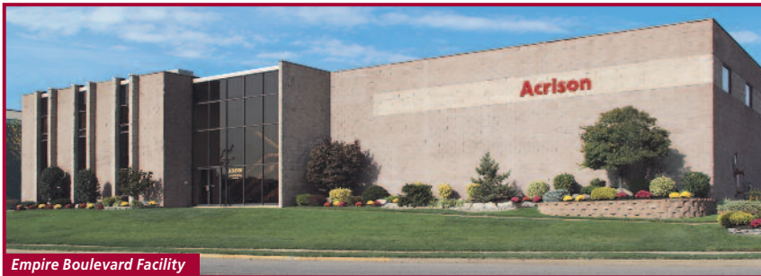
Empire Boulevard Facility Moonachie, NJ USA
