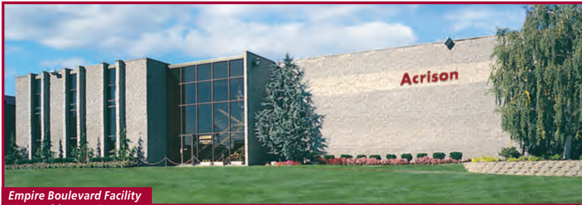
Empire Boulevard Facility Moonachie, NJ USA
