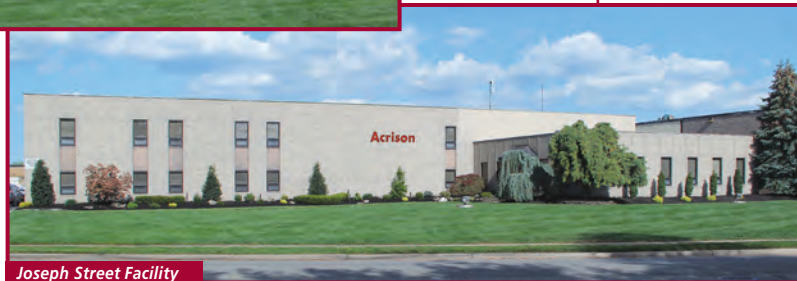
Joseph Street Facility Moonachie, NJ USA
