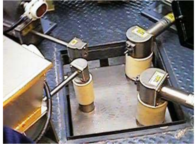
Four volumetric feeders discharge raw materials to a continuous blender, which feeds the mixture to an extruder. Operation is 7 days a week, 24 hours a day.
