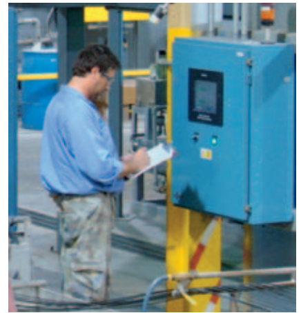
An operator checks feeder operation via the multifeder controller on one extrusion line.
