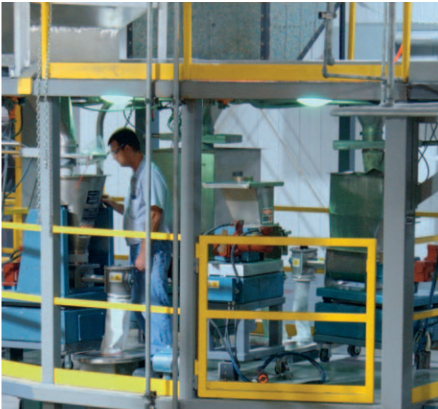
An operator stands among one extrusion line's various-sized gravimetric loss-in-weight feeders on the first-level mezzanine.
