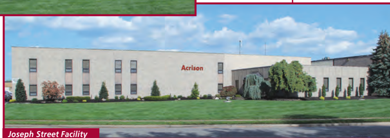
Joseph Street Facility Moonachie, NJ USA
