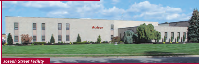
Joseph Street Facility Moonachie, NJ USA
