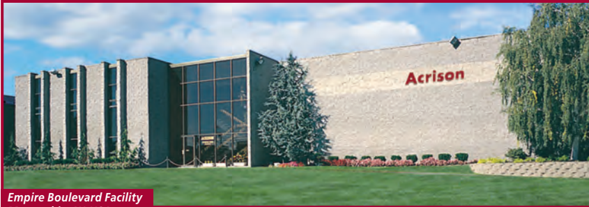
Empire Boulevard Facility Moonachie, NJ USA
