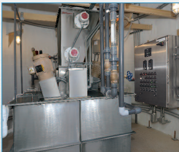
Equipment in this skirted silo includes several dry solids feeders metering chemical into dissolving tanks plus all required ancillary equipment and applicable controls.
