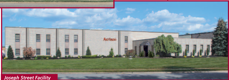
Joseph Street Facility Moonachie, NJ USA
