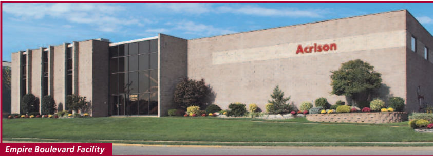
Empire Boulevard Facility Moonachie, NJ USA
